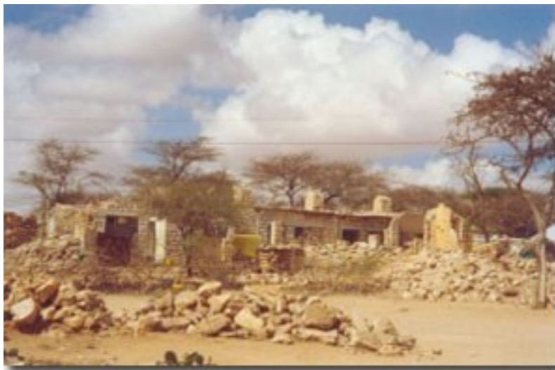
Edna's hospital destroyed by war.
